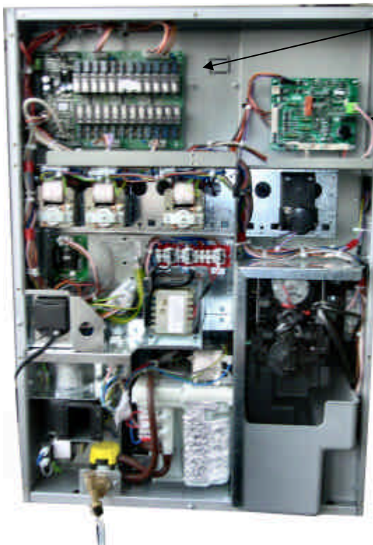
REAR SIDE WITHOUT CASING – LOCATION OF ACTUATION BOARD AND FRESH BREWER UNIT CONTROL BOARD
